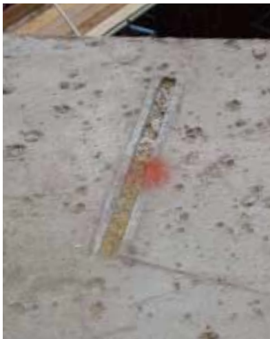
Facade connections using toothed HZA channels to provide adjustment in the direction of the wind load. One or two channels can be used per bracket.
