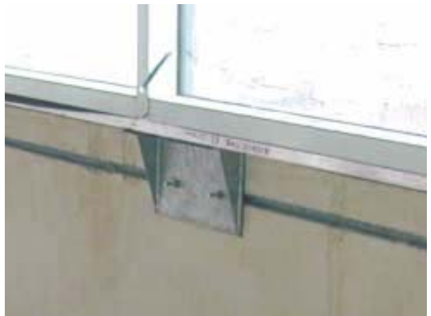
Typical window connection to precast panel.
