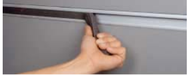
When concrete is set, remove the formwork, then remove the filler material from the channel.
