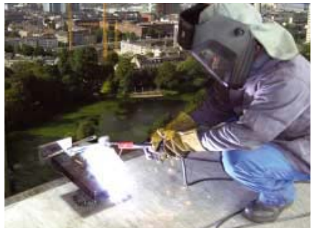
Welding requires difficult repositioning of heavy equipment and a costly energy supply.
