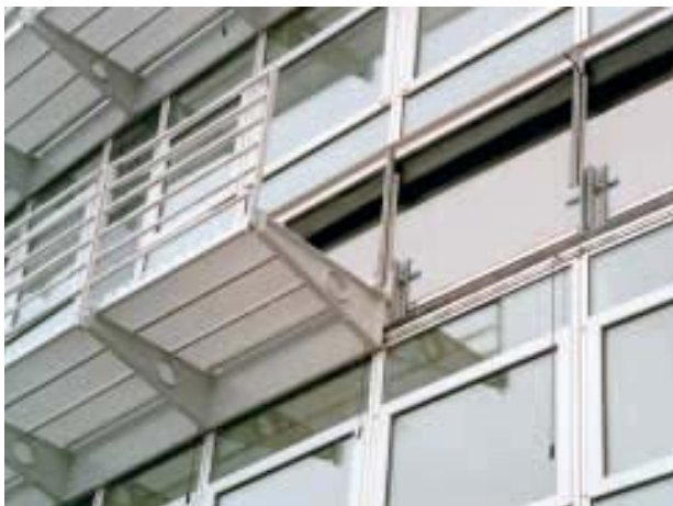
Sunscreen connections using channels to support vertical & horizontal loads.
