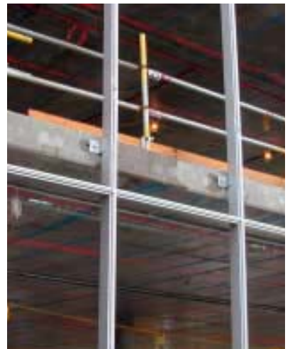
Typical connection to the edge of a post tensioned floor slab.
