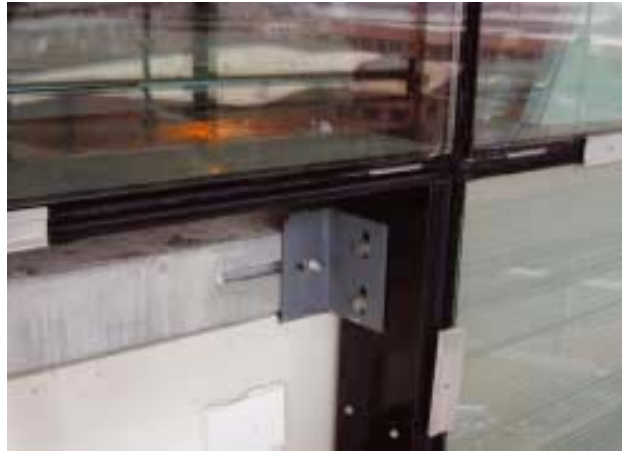
Typical facade connection to the edge of a floor slab.
