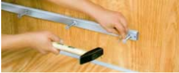
Nail channel to formwork
