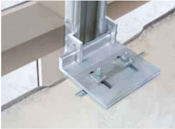
Typical facade connection to the top of floor slab.
