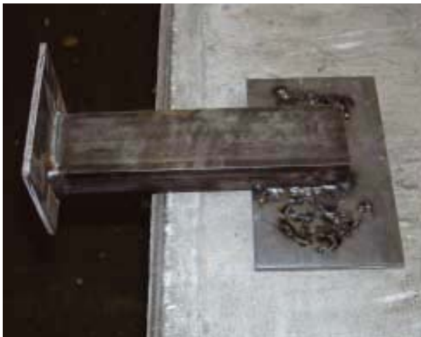
Weld and paint splatter can cause expensive damage to the facade.
